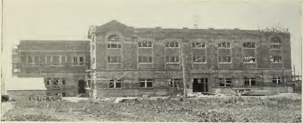
THE NEW MEN'S GYMNASIUM, UNFINISHED.
